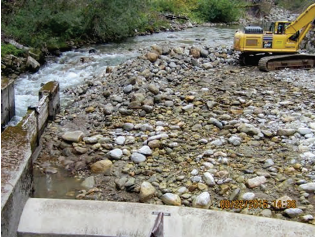
Figure 4.2-1. Intake pool area during cleanout.
