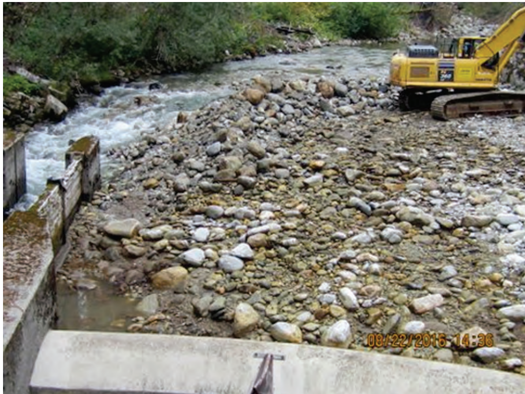
Figure 4.2-1. Intake pool area during cleanout.
