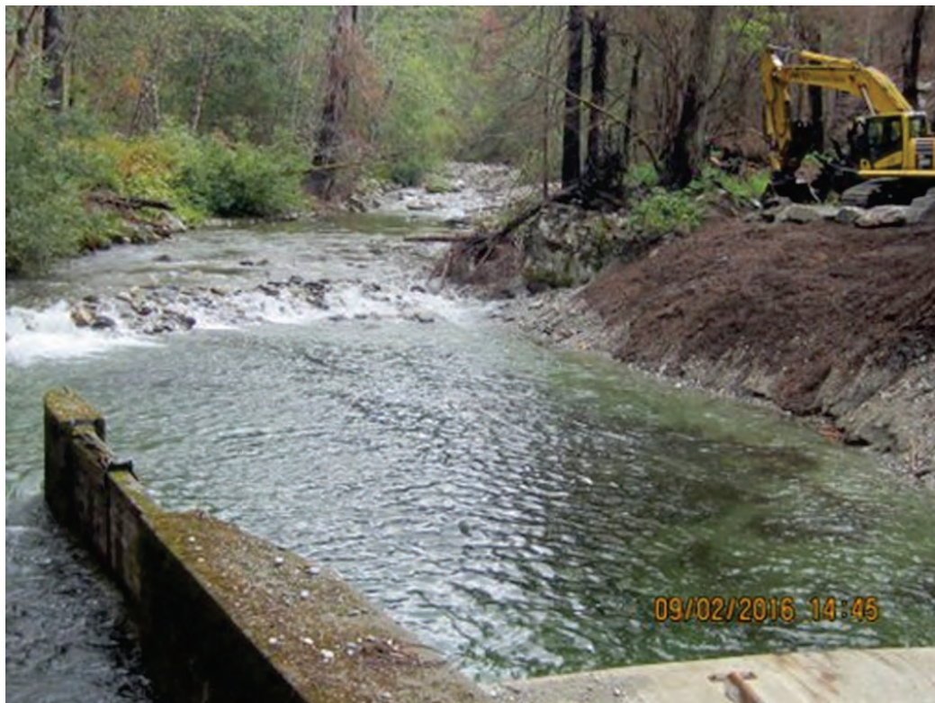
Figure 4.2-2. Intake pool following cleanout.
