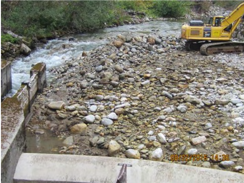
Figure 4.2-1. Intake pool area during cleanout.
