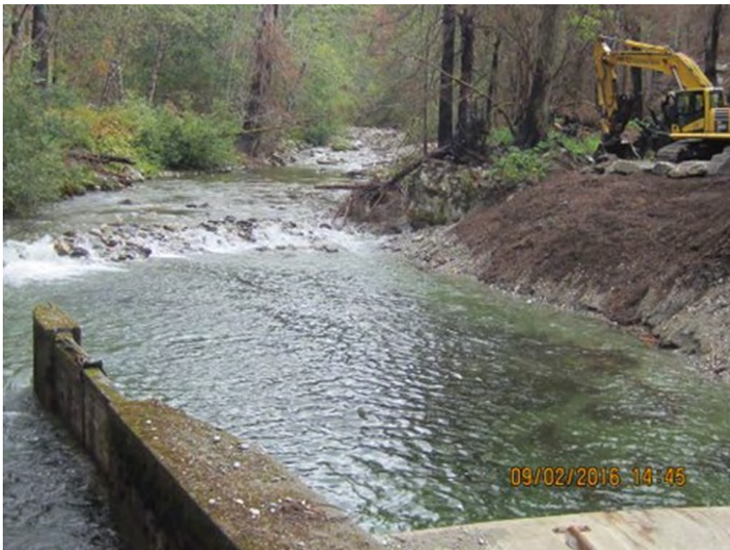
Figure 4.2-2. Intake pool following cleanout.
