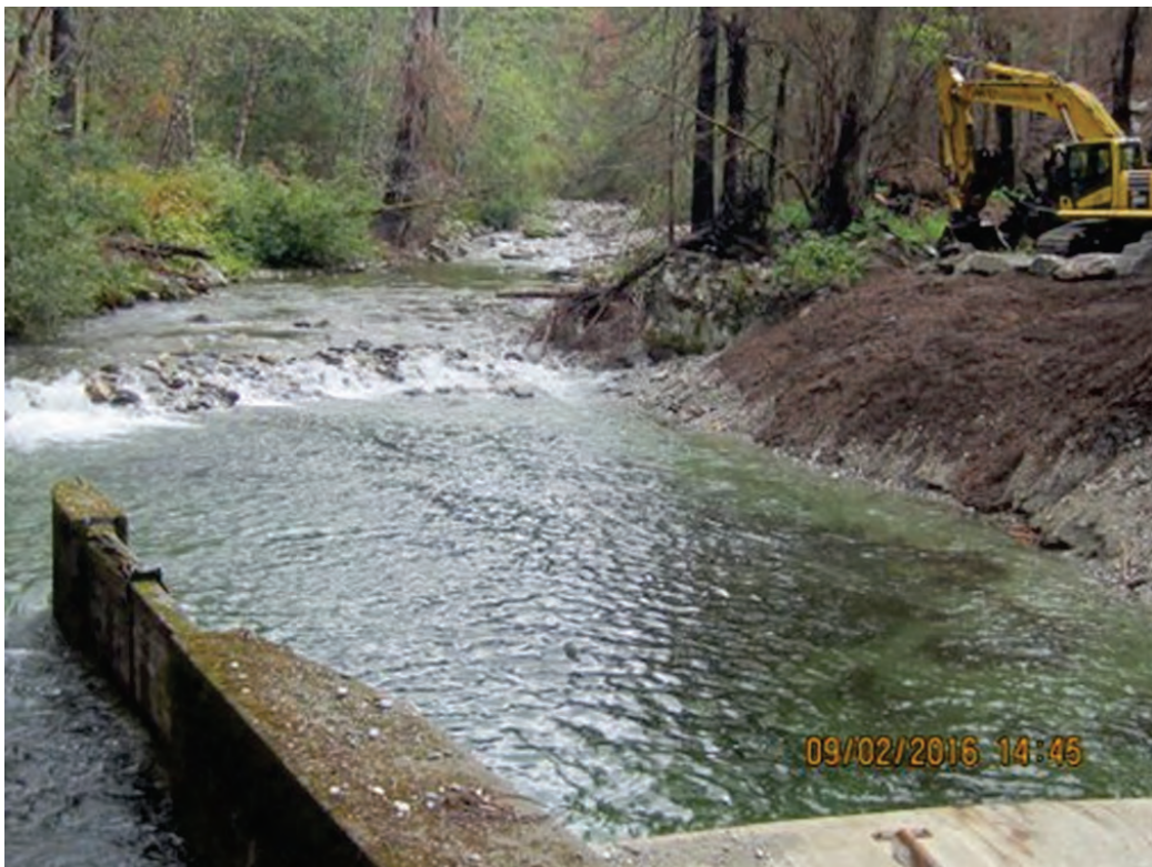
Figure 4.2-2. Intake pool following cleanout.
