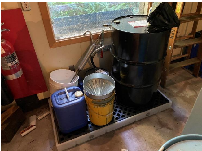
Photograph 17. Oil storage area in northern portion of powerhouse.
