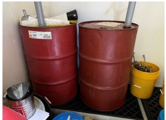
Photograph 18. Oil storage in shed south of powerhouse.
