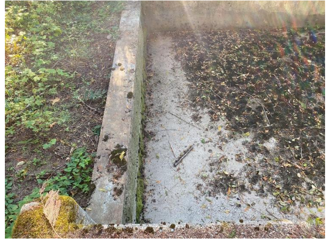
Photograph 200. Tailrace fish barrier located north of powerhouse.
