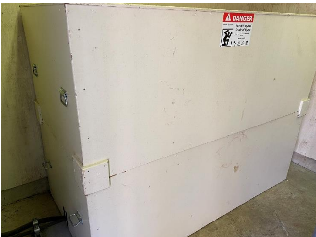
Photograph 5. Power tunnel access point.
