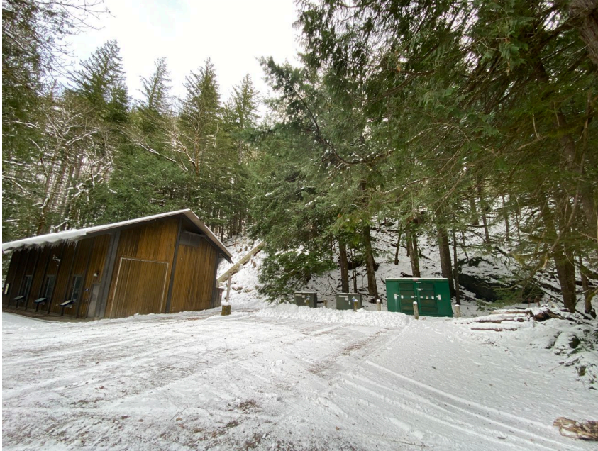
Photo 1. View of the three transformers associated with the Newhalem Creek powerhouse. The larger transformer (right) is air cooled.
