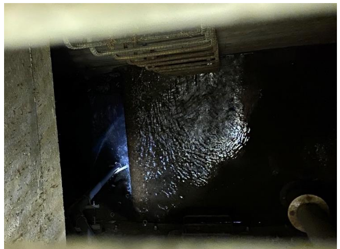
Photograph 6. Interior of power tunnel access point.
