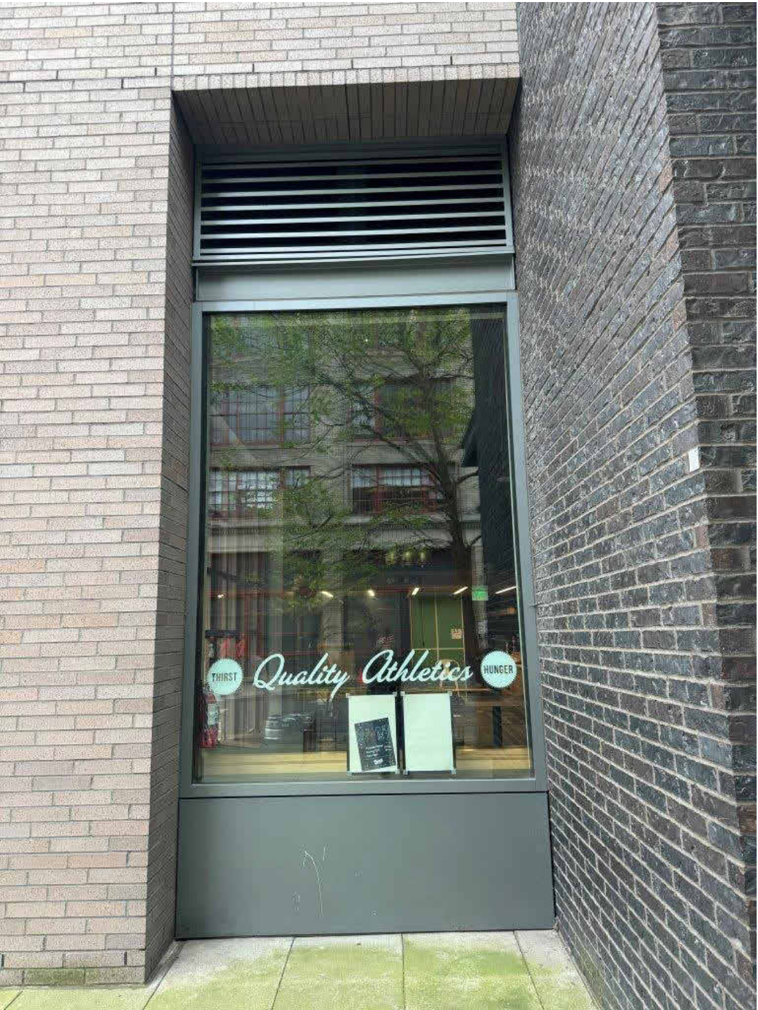
EXISTING STOREFRONT WHERE PROPOSED ENTRY DOOR IS LOCATED
