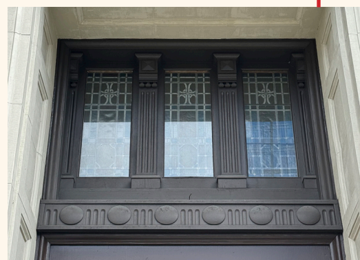
Detail of transom window featuring leaded glass and classical detailing
