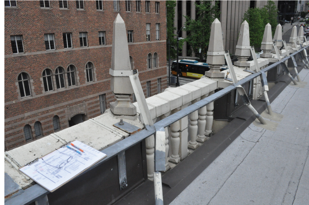
Figure 26: Finial and parapet bracing was installed in 1994. The bracing requires several repairs to comply with current code for parapet bracing requirements. 210526 PAC ROOF DSC_0875.JPG. Credit: Richaven, 2022
