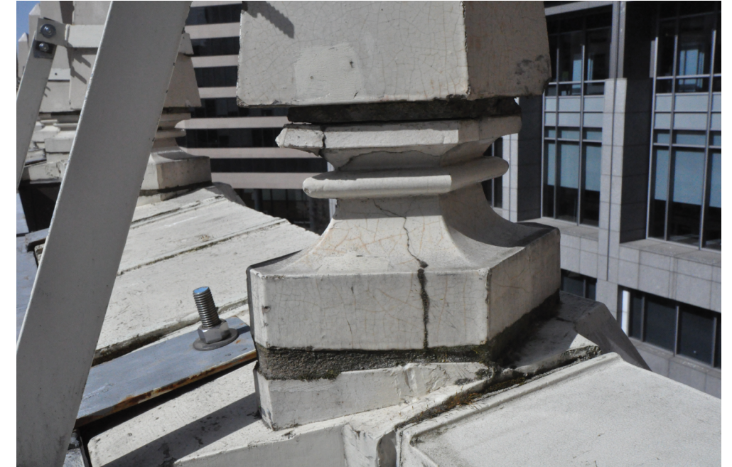
Figure 28: In several locations, original terra cotta blocks are cracking, spalled, or broken and are proposed to be replaced in-kind. See the color coded blocks on the building elevations. 210407 Pacific Hotel - DSC_0179.JPG. Credit: Richaven, 2022
