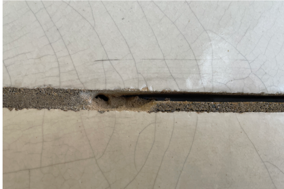
Figure 18: Typical crazed terra cotta and mortar joint at the Pacific Apartments. Note the soiled or skim coated mortar at the surface compared to the warm colored mortar deeper in the joint. 220222 PH-Pac Sample 10 IMG_1100.JPG. Credit: Richaven, 2022
