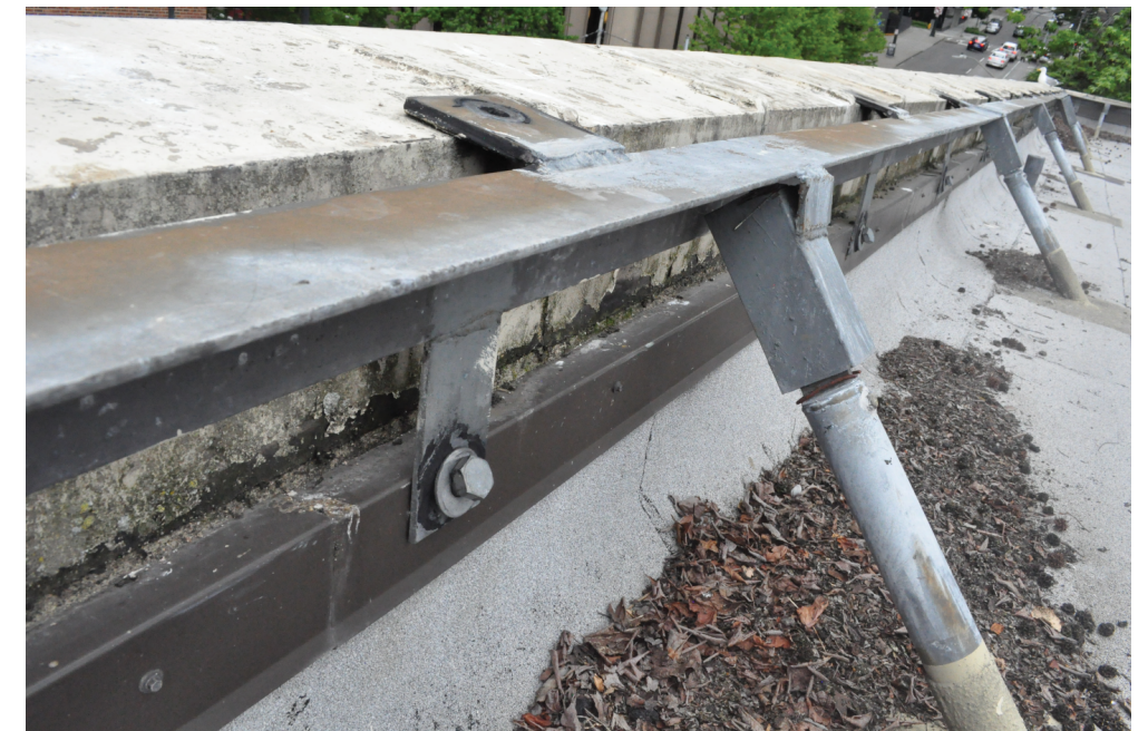
Figure 29: In some locations, parapet anchor bolts were not installed or were not sealed. Repairs are proposed to comply with current parapet bracing requirements. 210526 PAC ROOF DSC_0900.JPG. Credit: Richaven, 2022
