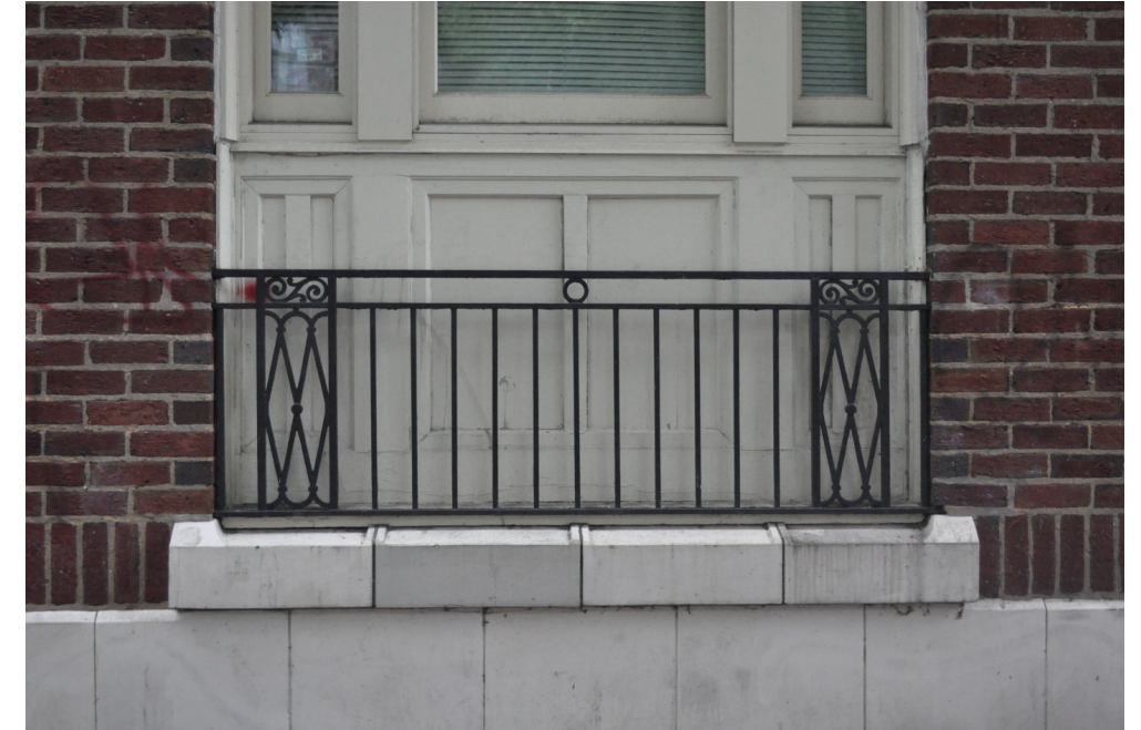
Figure 22: Typical historic wood wainscot at the base of the 2019 replacement windows illustrates minor wood repairs required, spray paint graffiti, and building soiling. 210526 PAC EL-E DSC_0648.JPG. Credit: Richaven, 2022
