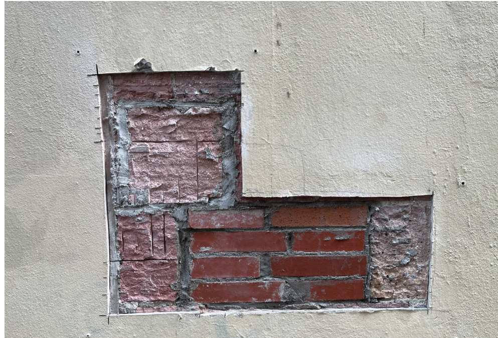
Figure 30: Samples of stucco cladding were removed from delaminated areas revealing multiple different substrates (clay tile, brick and concrete) and confirming no lath was originally installed. IMG_1305.JPG. Credit: Richaven, 2022
