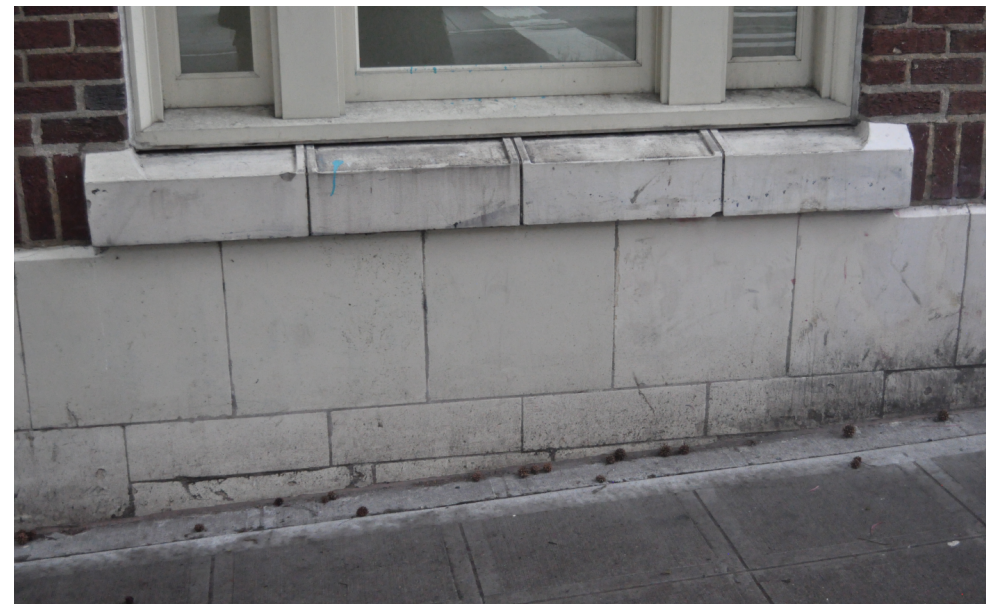
Figure 21: The terra cotta at the street level is significantly soiled with dirt, marker, paint, atmospheric soiling, backsplashed dirt, and other materials. 210526 PAC EL-E DSC_0651.JPG. Credit: Richaven, 2022
