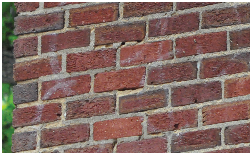
Figure 19: The brick and mortar at the northeast corner of the building illustrates the deterioration of the mortar and texture of the brick. Also present is the ghosted appearance of spray paint graffiti. 210526 PAC EL-N-E DSC_0479.JPG. Credit: Richaven, 2022
