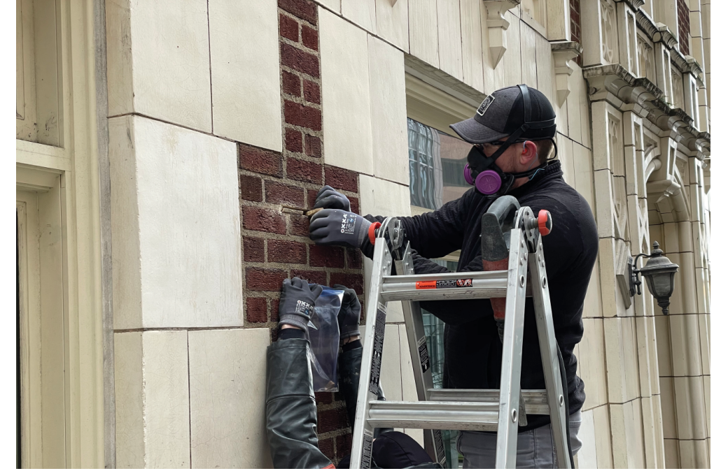
Figure 34: Mortar samples were taken at both brick and terra cotta for lab analysis to confirm the color, composition, and properties to be matched to ensure in-kind replacement materials. 220222 PH-Pac Sample 9 IMG_1091.JPG. Credit: Richaven, 2022
