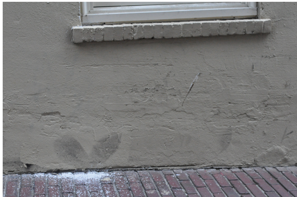
Figure 25: The west (alley) elevation of the building is coated in stucco directly applied to the hollow clay tile infill and reinforced concrete structure. This wall has been significantly damaged by vehicles and water damage and repaired multiple times. 210526 PAC EL-W DSC_0717.JPG. Credit: Richaven, 2022
