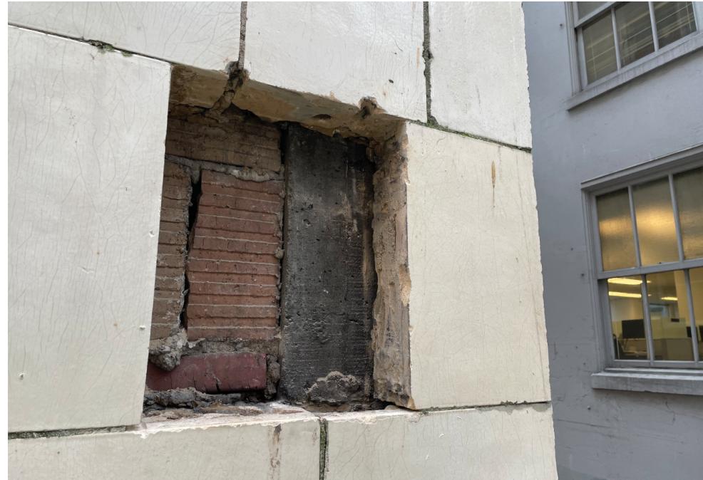
Figure 32: Terra cotta samples were removed where the existing materials were cracked or broken and planned to be replaced revealing multiple substrates and minimal anchoring of the masonry cladding. 220222 PH-Pac Sample 17 IMG_1261.JPG. Credit: Richaven, 2022
