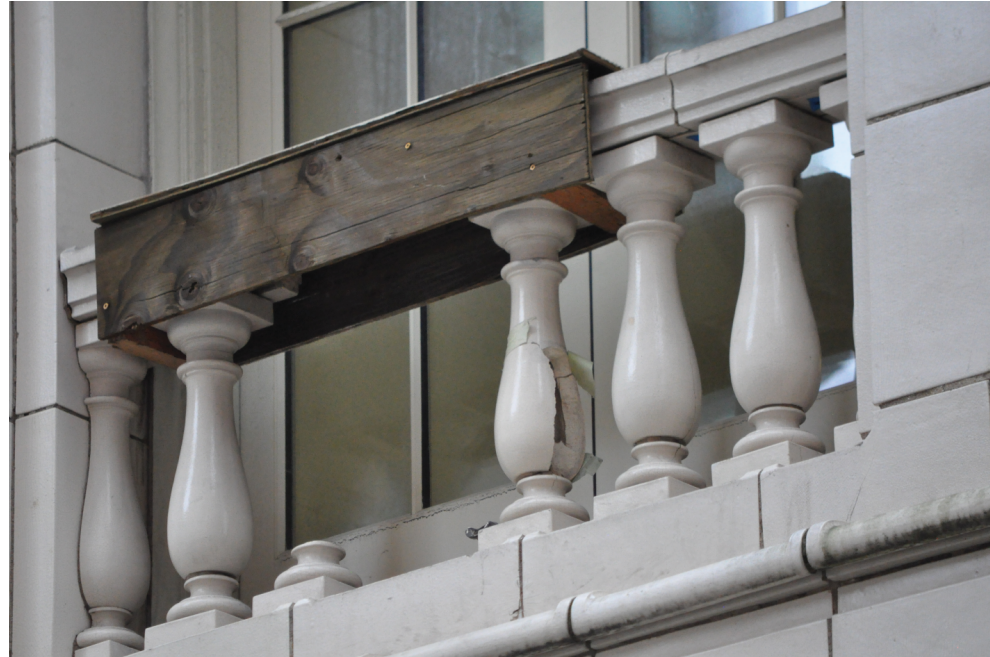
Figure 24: This severely deteriorated balustrade is located at the third floor level of the north elevation above the entry to the east (apartment) wing of the building. 210526 PAC EL-N-E DSC_0478.JPG. Credit: Richaven, 2022
