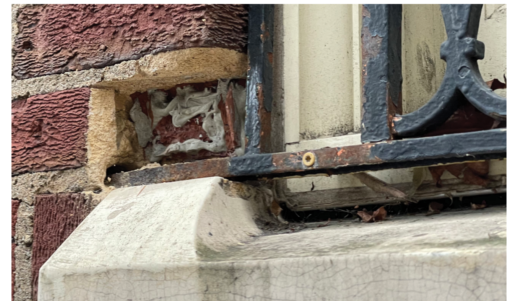
Figure 23: The brick at railings is often displaced, broken, or missing due to wear and tear on the railings, mortar deterioration, and rust jacking. Note the skim coat mortar patching over the yellow original mortar and the screw into the window. IMG_1051.JPG. Credit: Richaven, 2022
