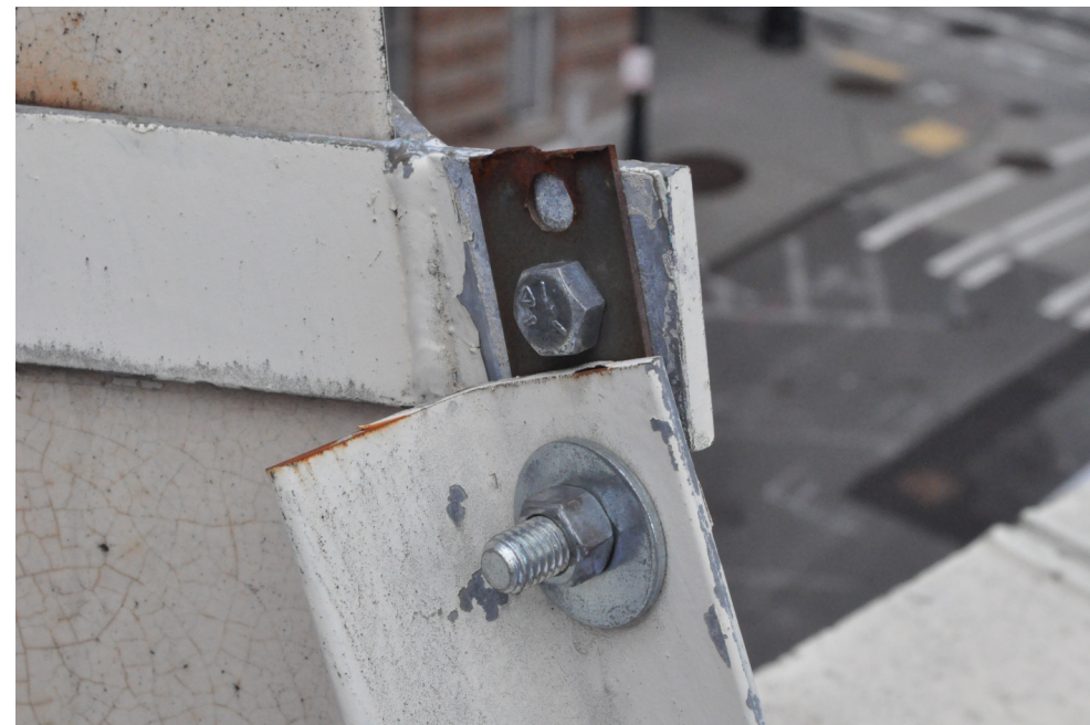
Figure 27: Make shift elements were added to the finial bracing to complete the original installation. Repairs are proposed to comply with current parapet bracing requirements. 210526 PAC ROOF DSC_0884.JPG. Credit: Richaven, 2022
