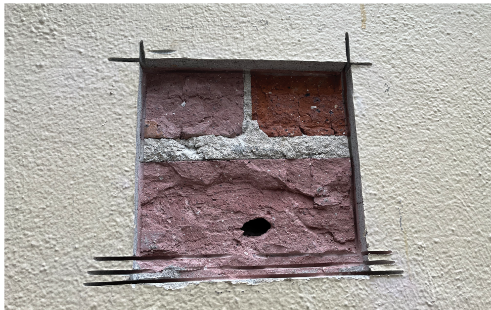
Figure 31: Stucco samples taken also revealed long term water damage to clay tile substrates where the cleavage plane was located in the thickness of the clay tile - not the stucco itself. 220222 PH-Pac Sample 12 IMG_1130.JPG. Credit: Richaven, 2022
