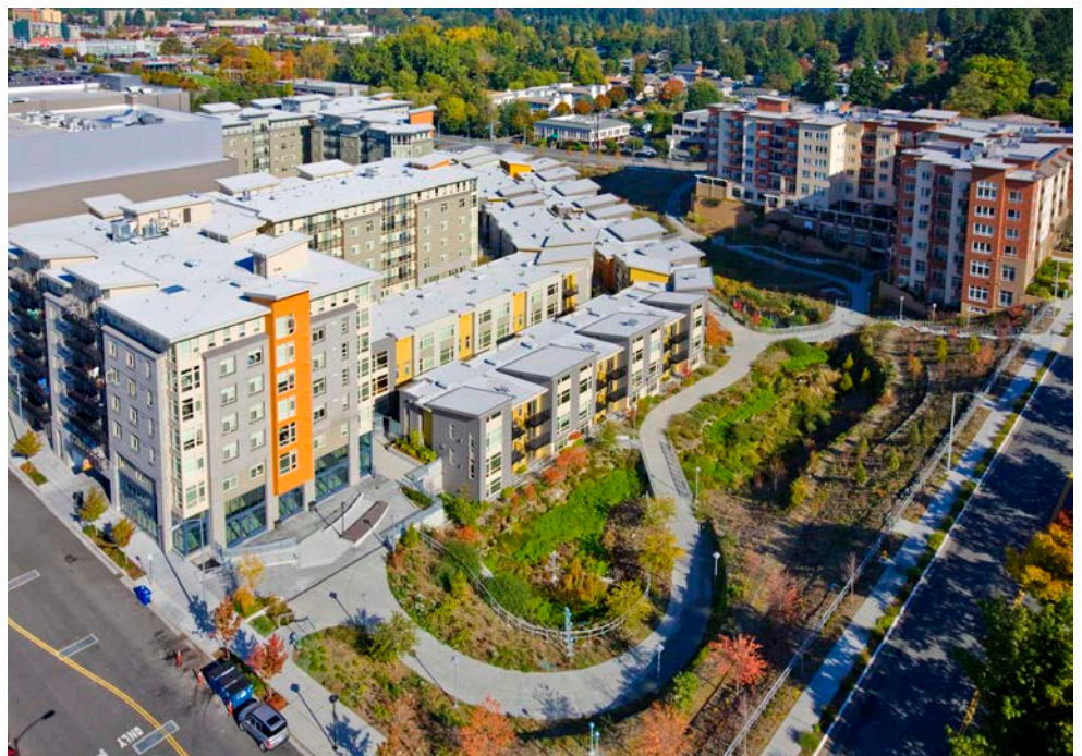
Thornton Creek Credit: MIG | SvR
