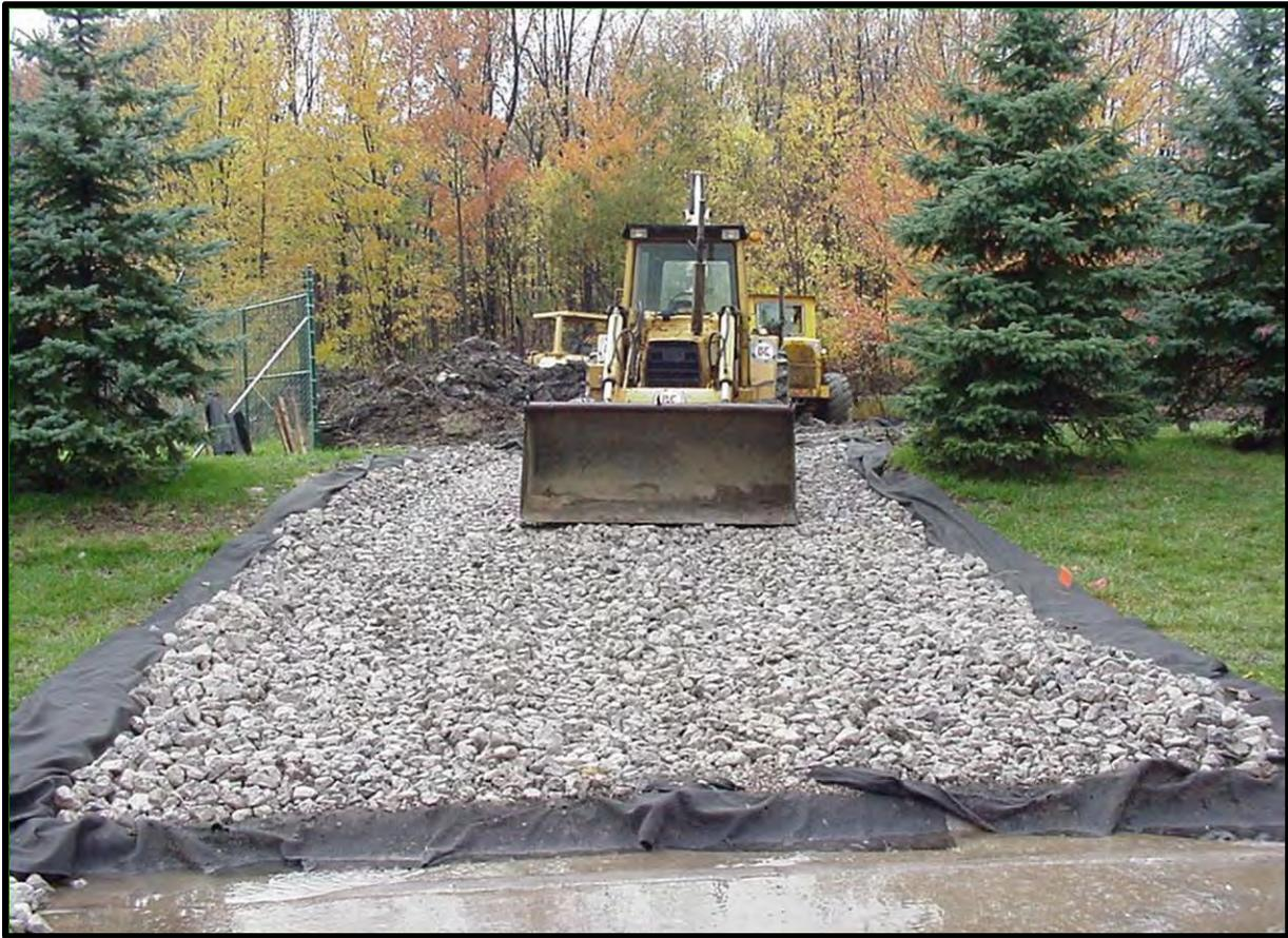
Figure 6. Stabilized Construction Access.
