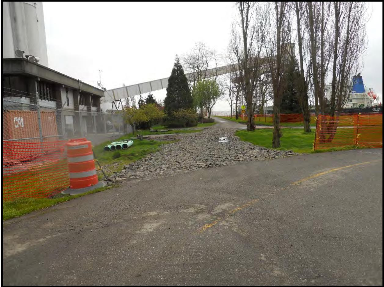
Figure 7. Stabilized Construction Access.
