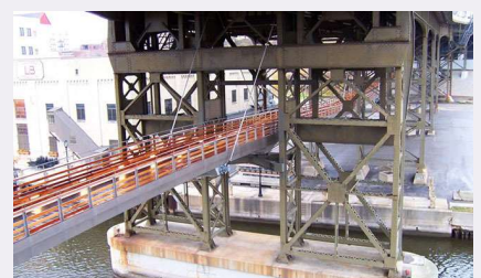
The Marsupial Bridge is a bike and pedestrian bridge supported by the existing vehicle bridge structure that creates direct pedestrian connection to a multi-use path network., .
