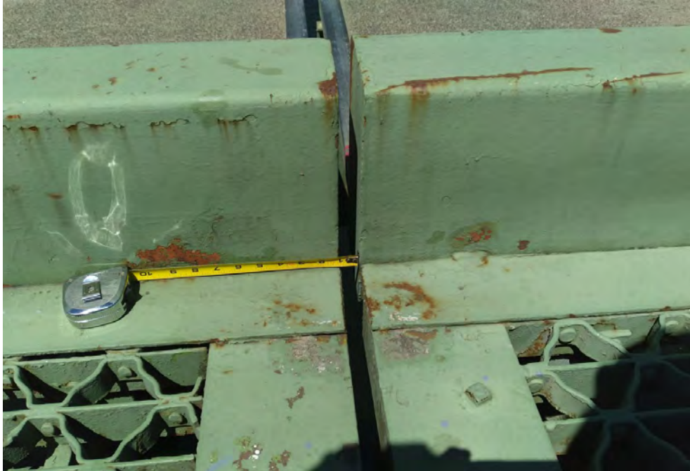
Figure 6. Limited gap between bascule leaves
