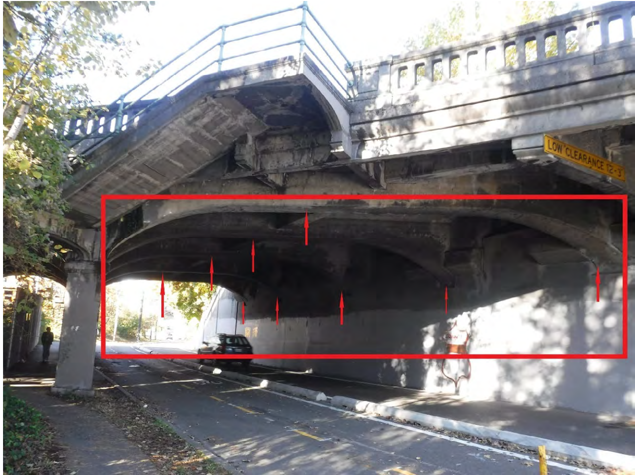
Figure 4. North approach, underside of east side of approach, looking west from NE 40th street. Ribbing and arches highlighted. Also note configuration of stairway (photo by HDR 2023).
