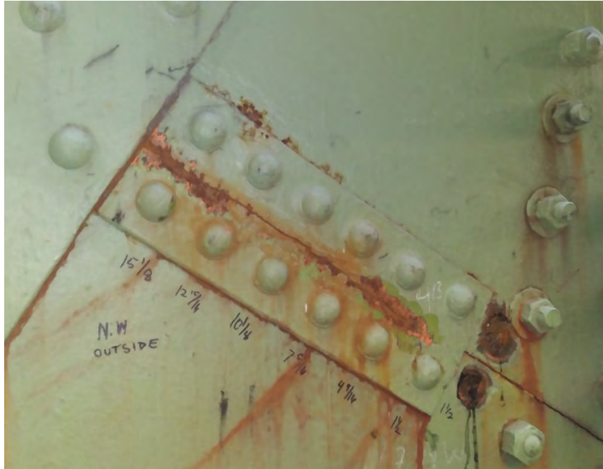
Figure 3. Cracked rack splice plate
