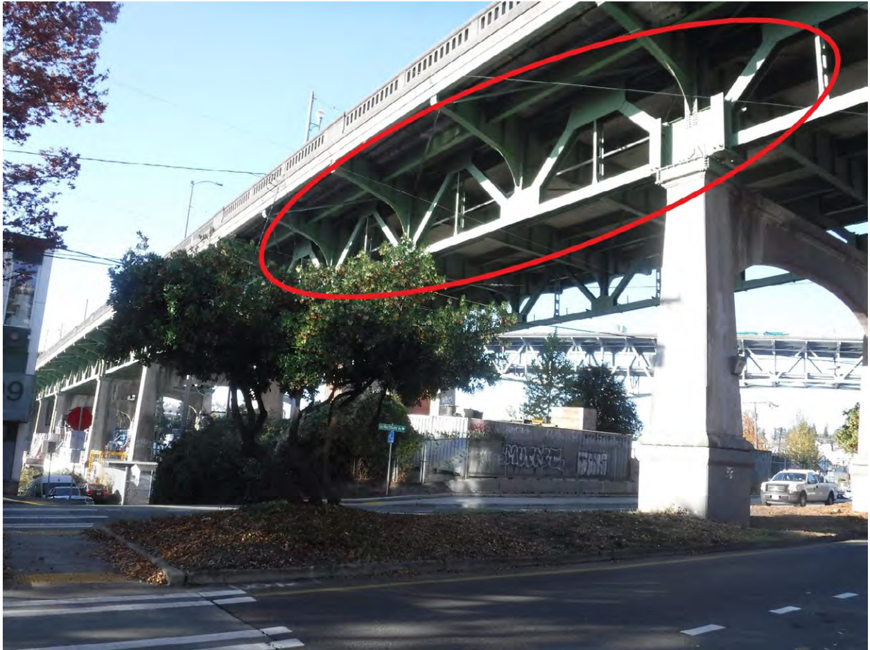
Figure 12. North approach looking northwest from NE Pacific Street, steel deck trusses highlighted in red (photo by HDR 2023).
