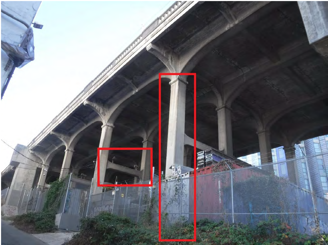
Figure 1. North Approach, underside of bridge deck, looking northeast. Concrete piers and "H" beams highlighted in red (photo by HDR 2023).
