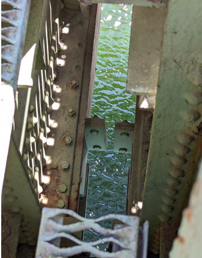
Figure 7. Steel angle and plates to be trimmed below the center lock
