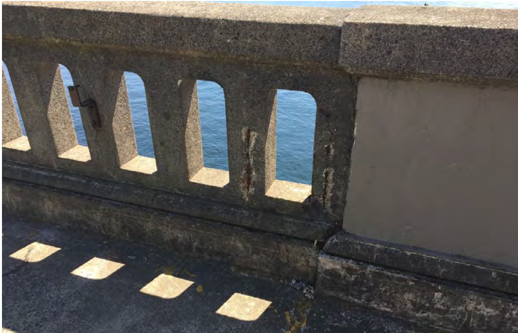
Figure 11. Concrete railing damage, typical
