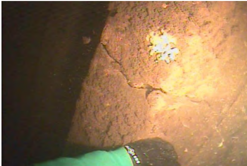
Figure 2. Typical pier cracks at Pier 3 (Source: 2018 UW inspection report)
