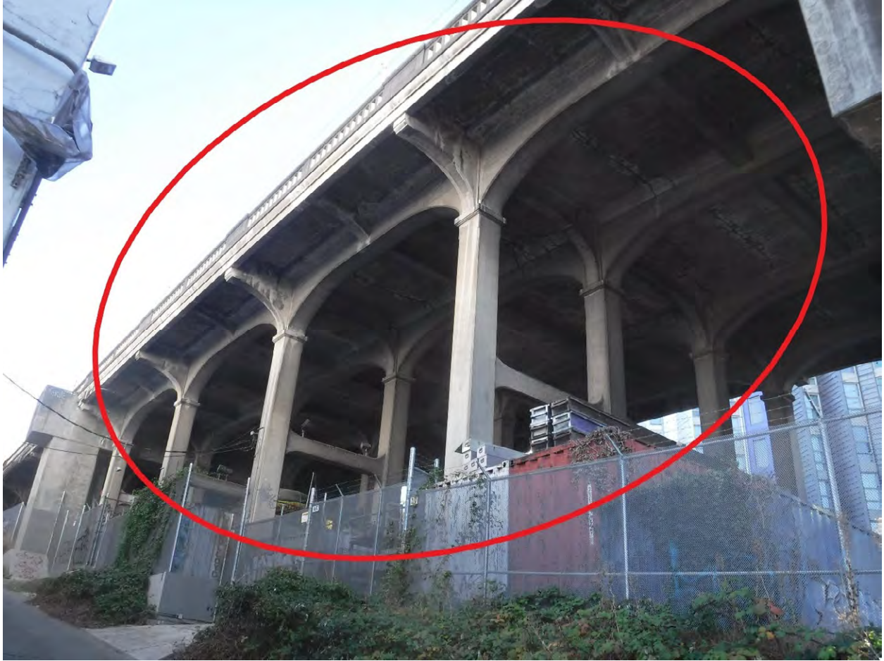
Figure 9. North approach, underside of deck looking northeast, overview of ribbing configuration highlighted in red (photo by HDR 2023).
