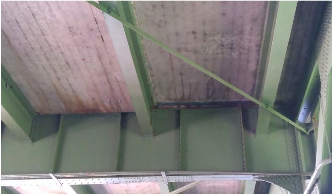
Figure 1. Water seepage and corrosion at south approach floorbeam
