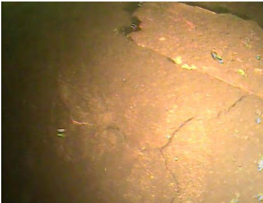
Figure 9. Pier column cracking (Source: 2018 UW Inspection Report)
