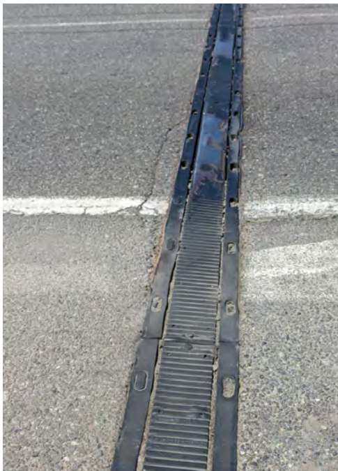
Figure 10. Expansion joint, typical
