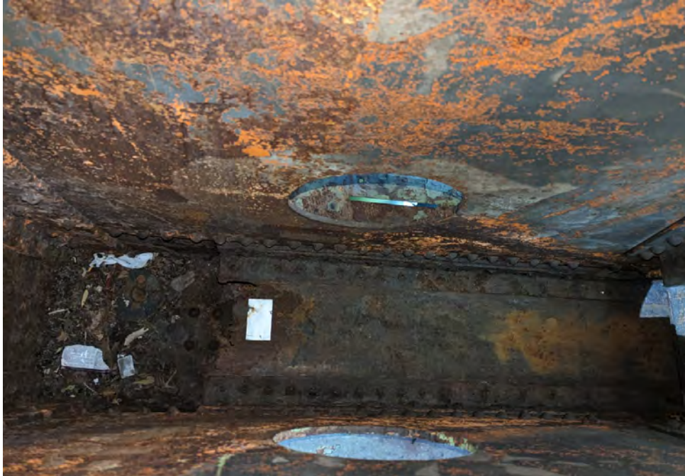
Figure 5. Corroded bottom chord (L7-L9)
