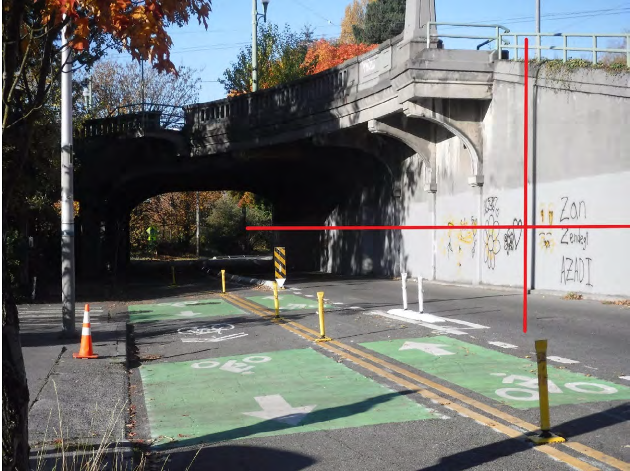
Figure 11. North approach, abutment looking west from NE 40th Street, configuration of abutment highlighted in red. Note that the sidewalk runs along the east edge of the abutment from the deck of the approach to NE 40th Street (photo by HDR 2023).
