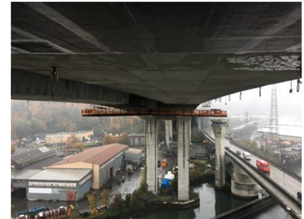
Temporary work platforms enable crews to do important stabilization work on the West Seattle High-Rise Bridge, and offer a unique view of the Low Bridge.
