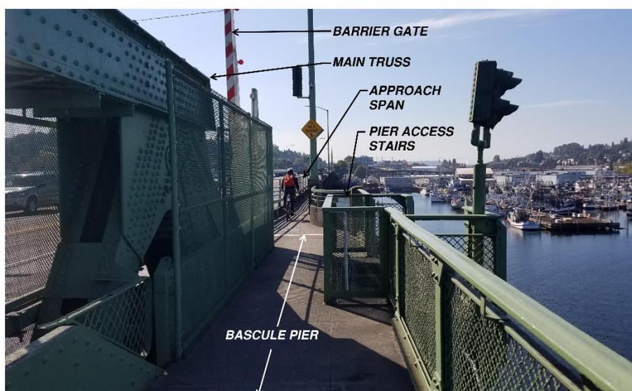
Figure 3. Existing Sidewalk at the Bascule Pier
