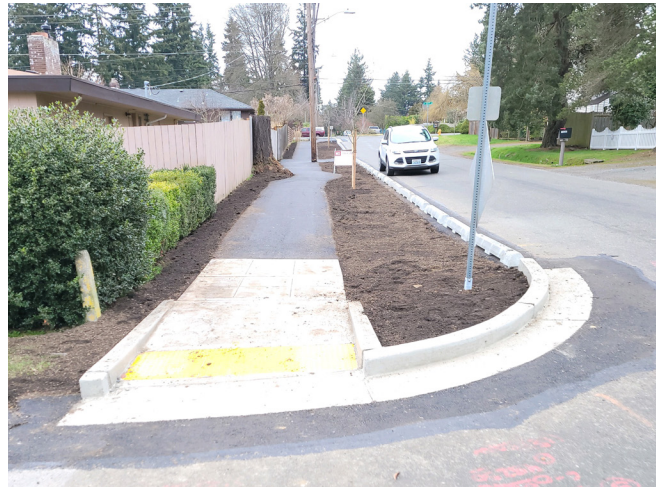
Walkway improvement on Ashworth Ave N for Ingraham High School
