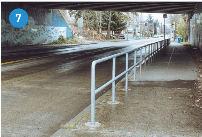
Handrail on S Cloverdale St under the Highway 99 overpass
