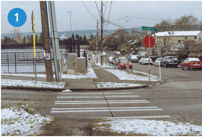
Cost effective walkway on 13th Ave S
