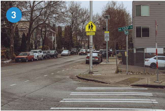
School zone flashing beacons on 35th Ave NE
