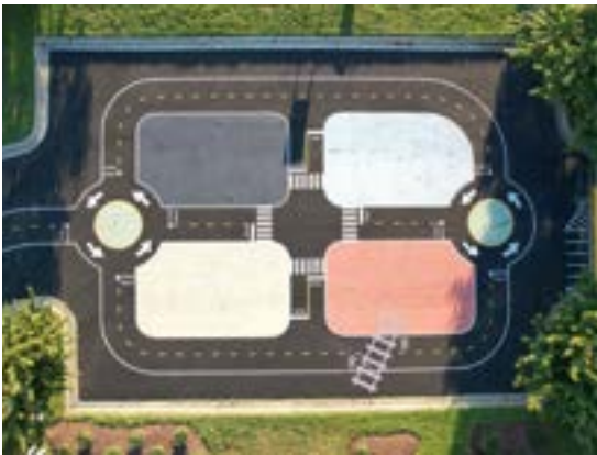
Seven Oaks Traffic Garden, MD: Existing closed-off parking lot next to open recreational area.
