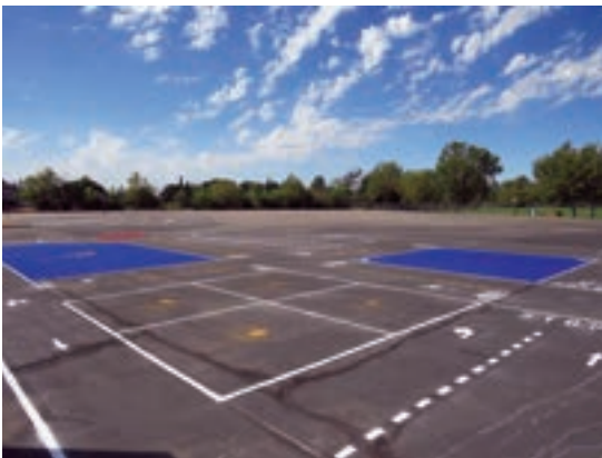
Auburn Elementary Traffic Garden, CA: The interior spaces serve as four-square courts.
