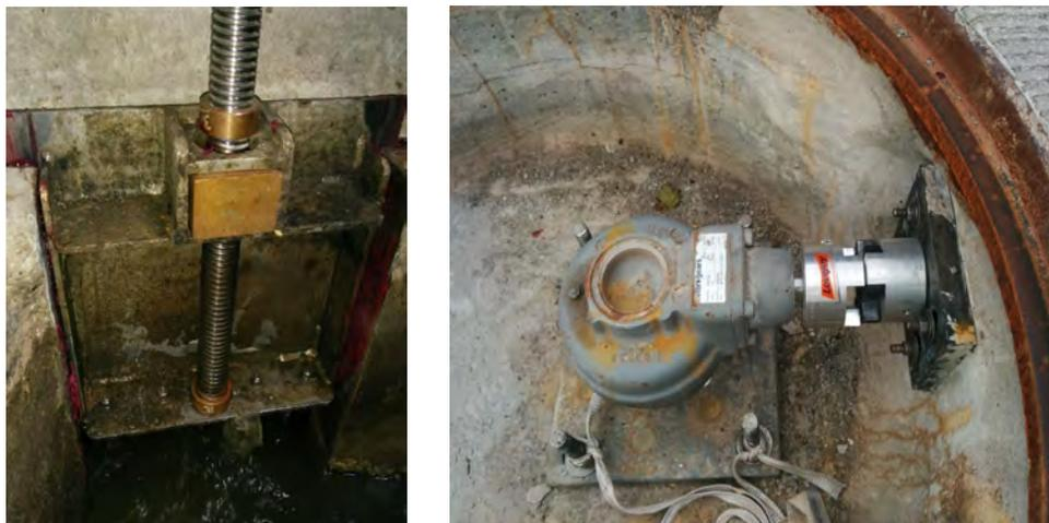
**Figure 4-1. New Basin 99 Sluice Gate (left) and Actuator Motor (right)**
