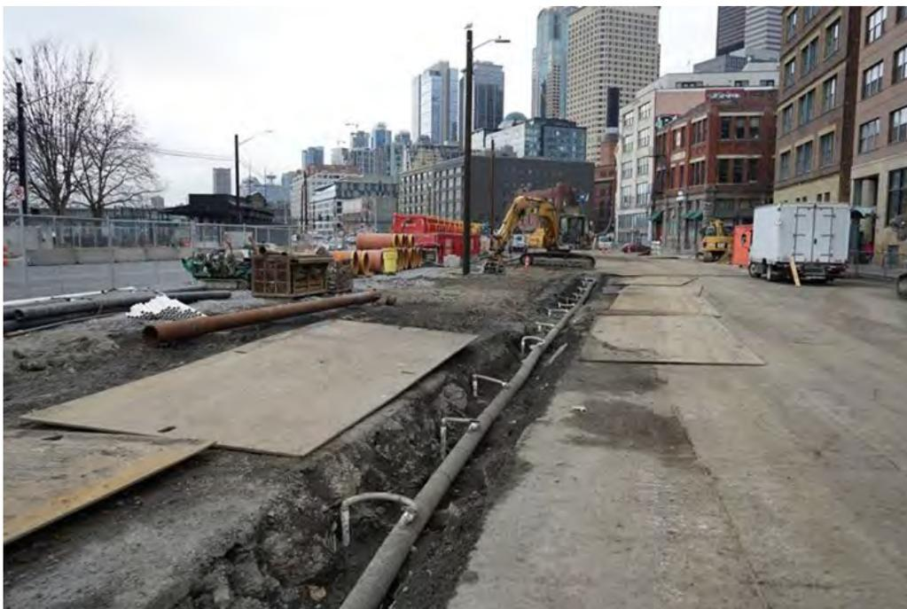
**Figure 4-7. Central Waterfront Construction – Dewatering System**
