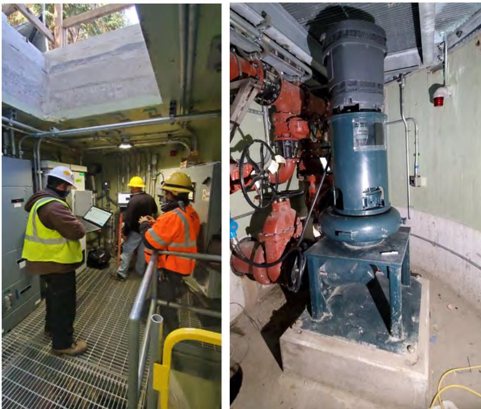
**Figure 4-3. Operational Testing of Upgraded Pump Station 13 (left) and new pumps and valving (right)**
