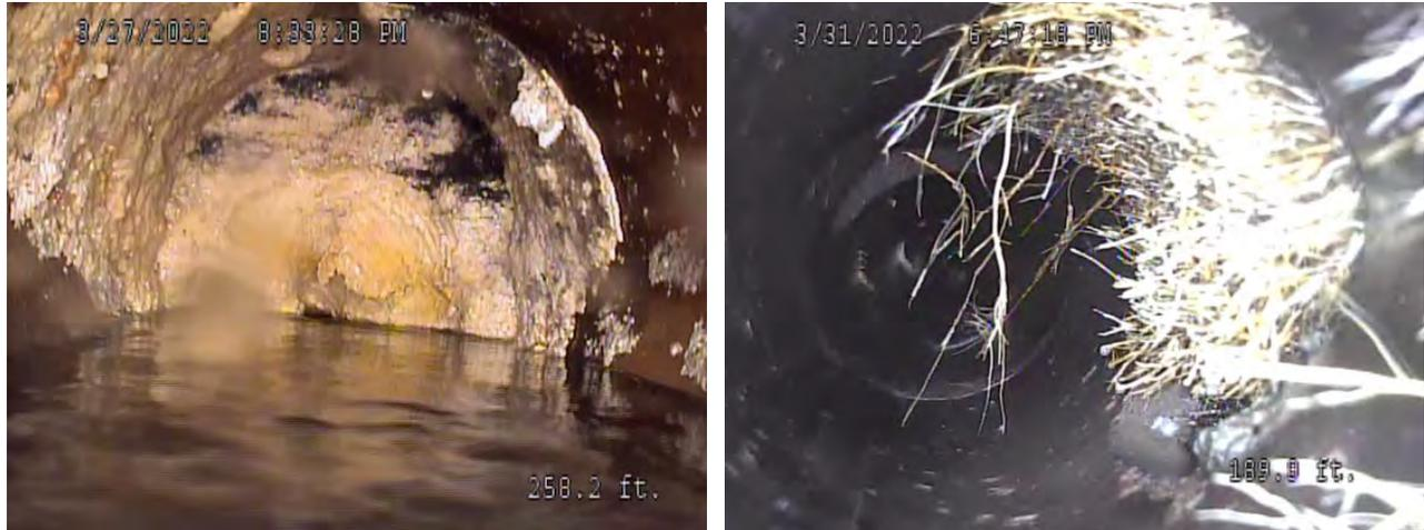
**Figure 3-2. 2022 Private side sewer connections demonstrating visible FOG accumulations and impacts from root intrusion**
